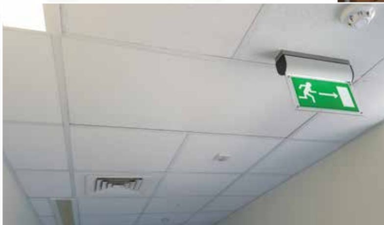
Radiant ceiling panel providing an almost invisible source of heat in a hospital corridor
